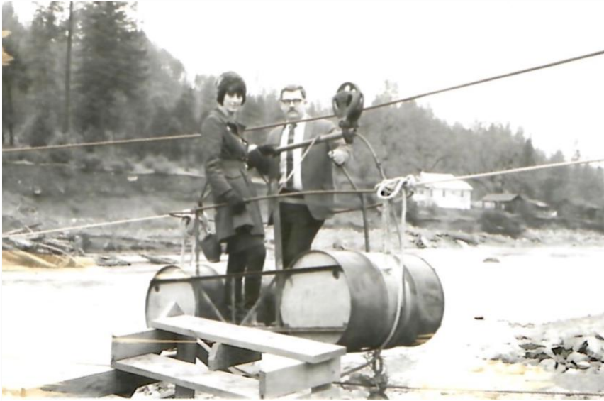
Teachers Leon, and Susan Spiegel on the temporary cable system to get to school over the river until a new bridge could be built. 1970
